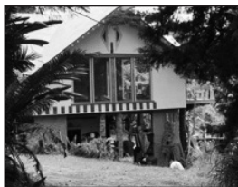
Footprints Classroom Building
